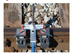
Insert Cadweld Plus cup into mold.
